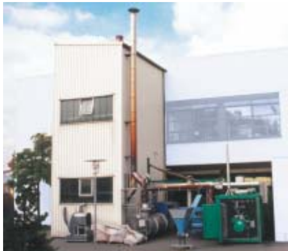
Figure 2: 0.5 MW-pilot plant in Oberhausen; left side: gasifier building, right side: drying plant and BHPP with gas engine
